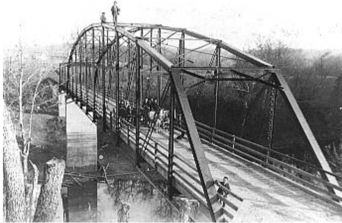
The 1904 Highway 12 bridge once spanned the White River. Today a 1963 bridge has taken its place. (Neg. #N009159)
